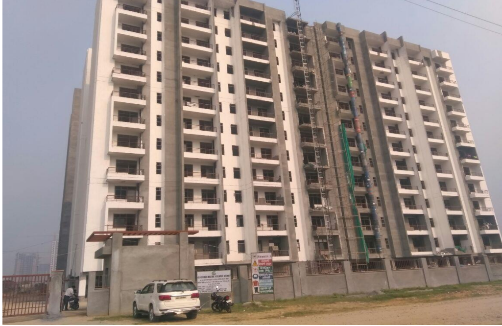
3BHK ( Area 132.95 Sqm) Photograph : as on 25-10-2017
